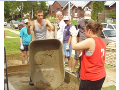
-Members from our group building a wheelchair ramp. Great work!
